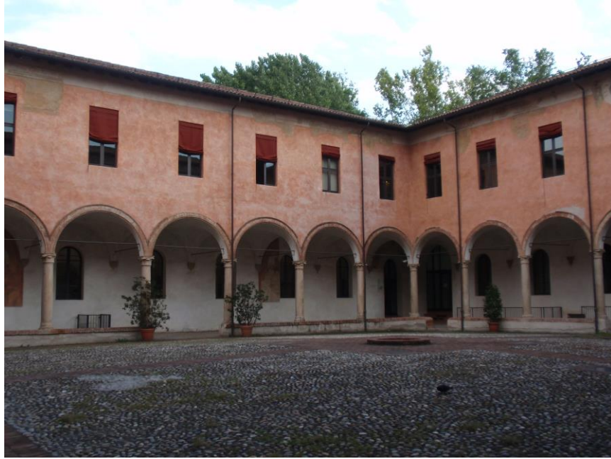
Figure 1: View into the courtyard of Santa Cristina as it appeared in 2010. The windows under the arcade on the left look into what used to be the common and laundry rooms. The space is now a women's studies library.
