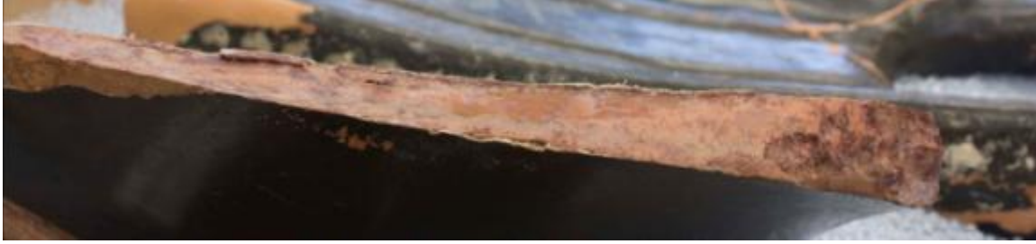
During Treatment after removal of third application. Total time elapsed = 1 hour 40 minutes
