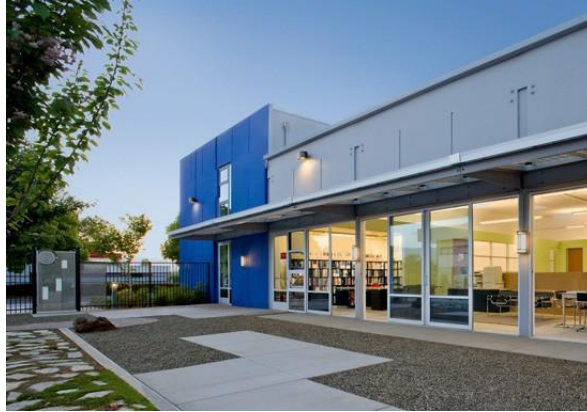
Figure 4.1. Integral Group office building exterior
