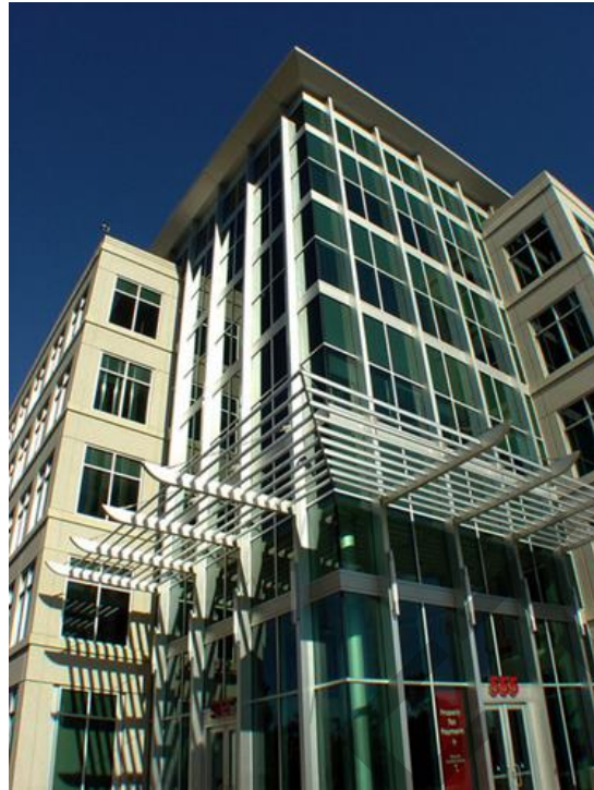
Figure 2.1. San Mateo County office building, Redwood City
