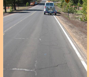
Structural assessment prior to action
