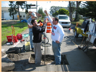
In pit DCP measurements
