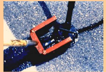
Crack seal
