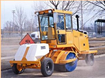
Brooming excess chip seal stone
