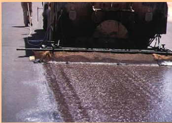
Slurry sealing
