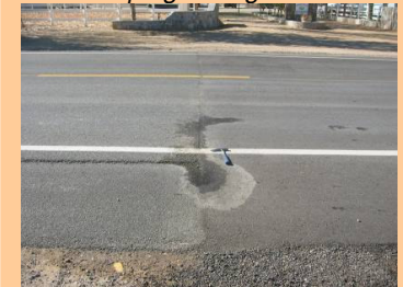
Pumping through patch joint
