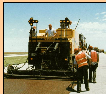
Microsurfacing application
