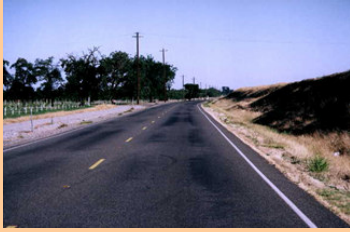
Failure criteria - bleeding
