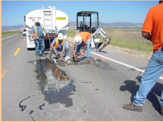
Saw cutting test pit
