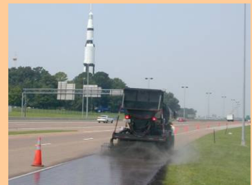
Shoulder fog seal
