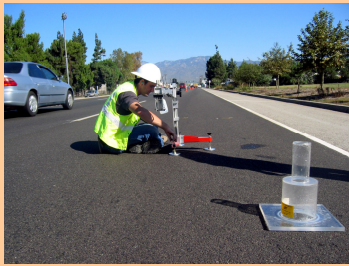
Skid resistance and permeability measurements
