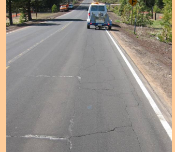
Structural assessment prior to action
