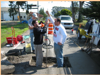
In pit DCP measurements
