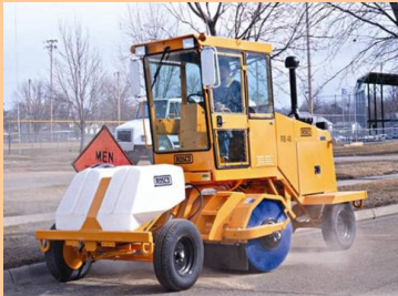
Brooming excess chip seal stone
