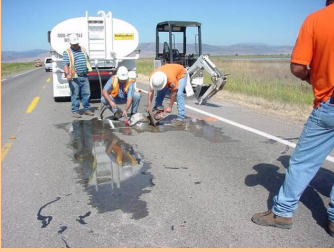
Saw cutting test pit
