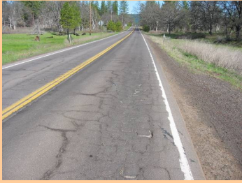
Consistent cracking
