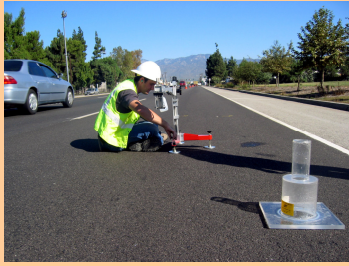
Skid resistance and permeability measurements
