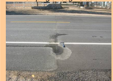
Pumping through patch joint
