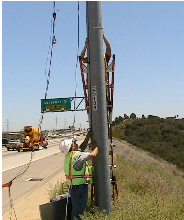
Figure 15 Two-Person Setup, Step 4: Tightening Top Pole Clamp
