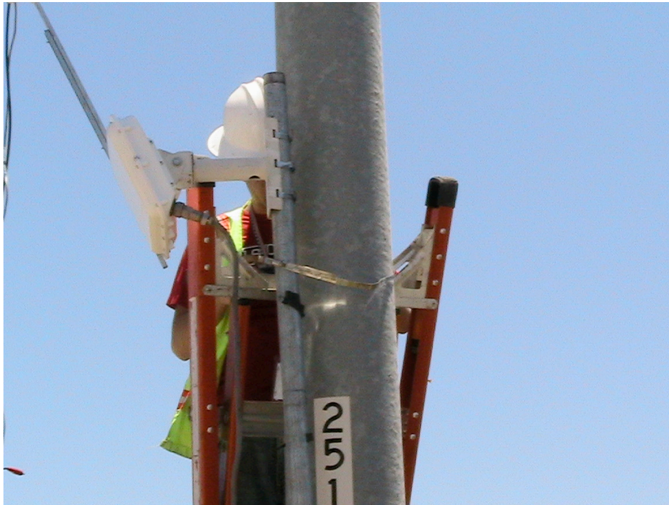
Figure 14 Two Person Setup, Step 4: Sliding Pole Up
