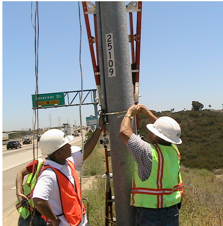
Figure 16 Two-Person Setup, Step 5: Tightening Bottom Pole Clamp
