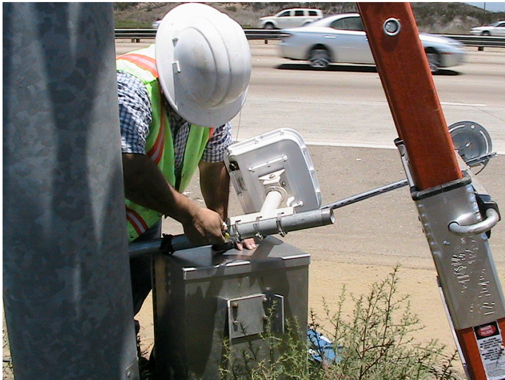
Figure 12 Two-Person Setup, Step 1: Attaching Sensor Assembly
