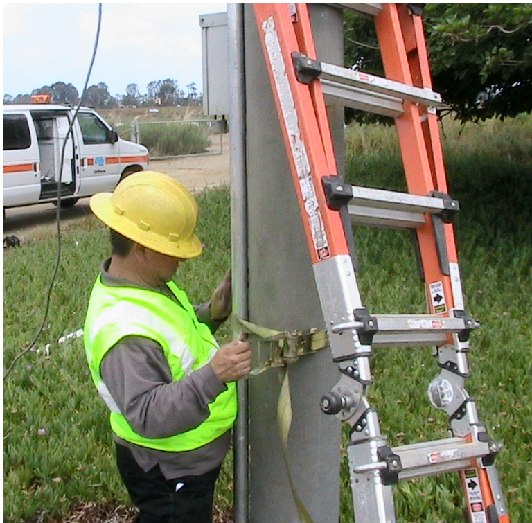
Figure 20 One-Person Setup, Step 5: Attaching Ratcheting Tie Down
