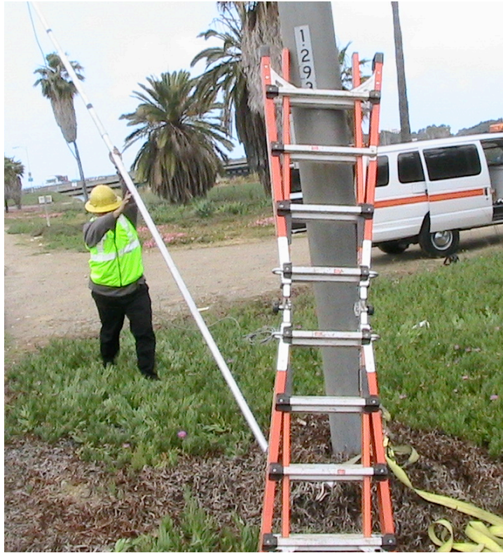
Figure 20 One-Person Setup, Step 5: Attaching Ratcheting Tie Down
