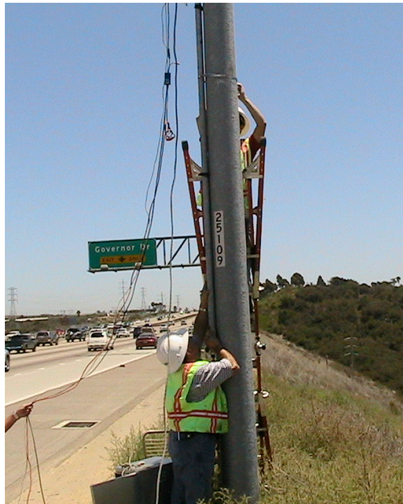
Figure 14 Two Person Setup, Step 4: Sliding Pole Up
