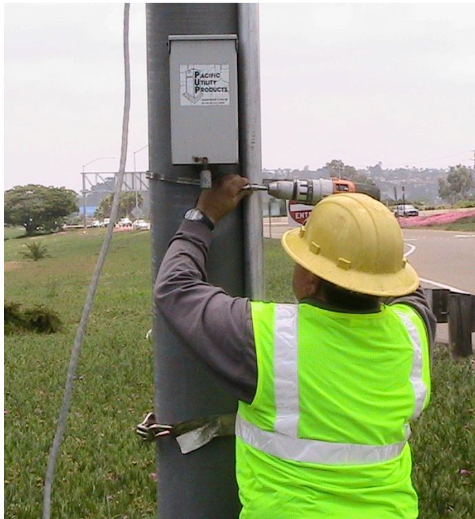
Figure 22 One-Person Setup, Step 7: Tightening Bottom Clamp
