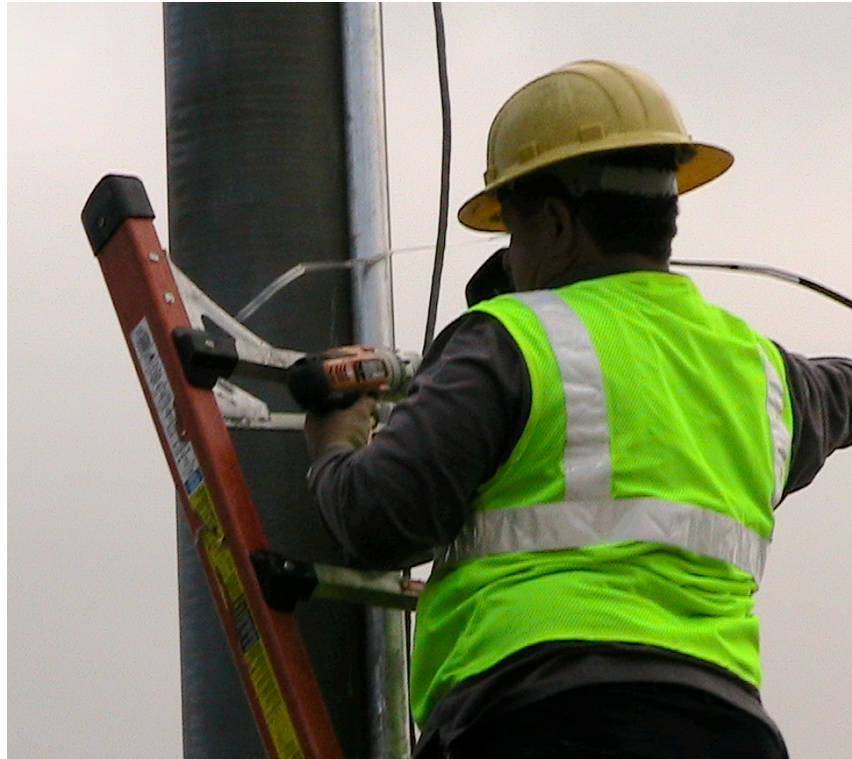
Figure 25 One-Person Teardown, Step 6: Removing Bottom Clamp
