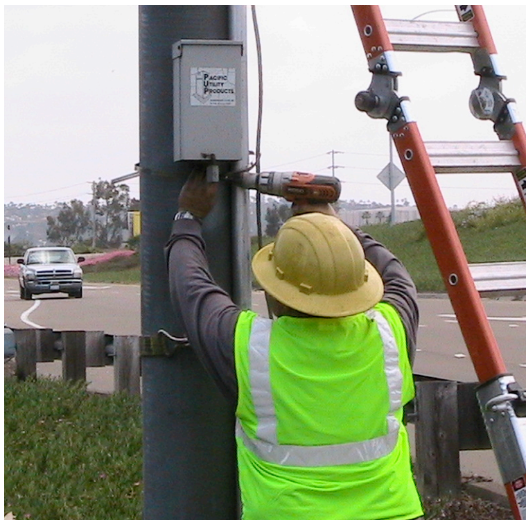
Figure 25 One-Person Teardown, Step 6: Removing Bottom Clamp
