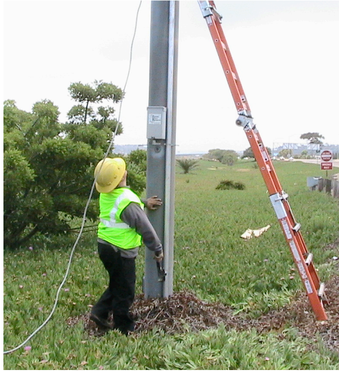
Figure 23 One-Person Setup, Step 9: Rotating Pole
