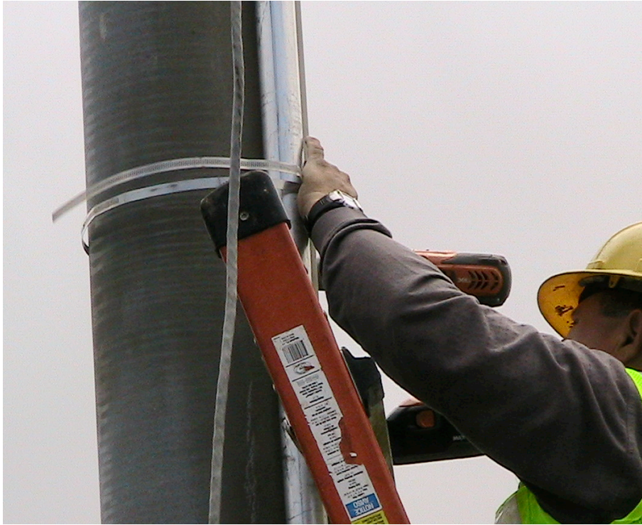
Figure 22 One-Person Setup, Step 7: Tightening Bottom Clamp
