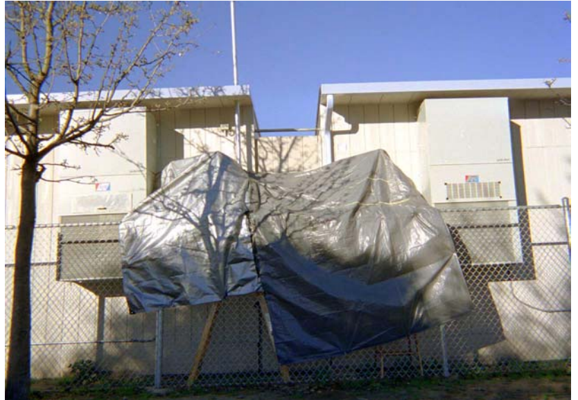
Figure 9 (a-d): LBNL designed rain protection for areas around the RC A outdoor enclosures during the winter 2002 heating season (a-b, CUSD, and c, MCS) and a special removable shelf for CUSD (d) to protect equipment and allow LBNL technicians to conduct field tasks regardless of ambient conditions or time of day.
