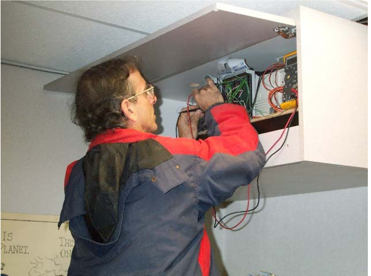
Figure 8a: Photographs of the completed (a) LBNL designed indoor cabinet (constructed for AMS and LBNL by Sierra Cabinets, CA for environment monitoring and computer equipment).
