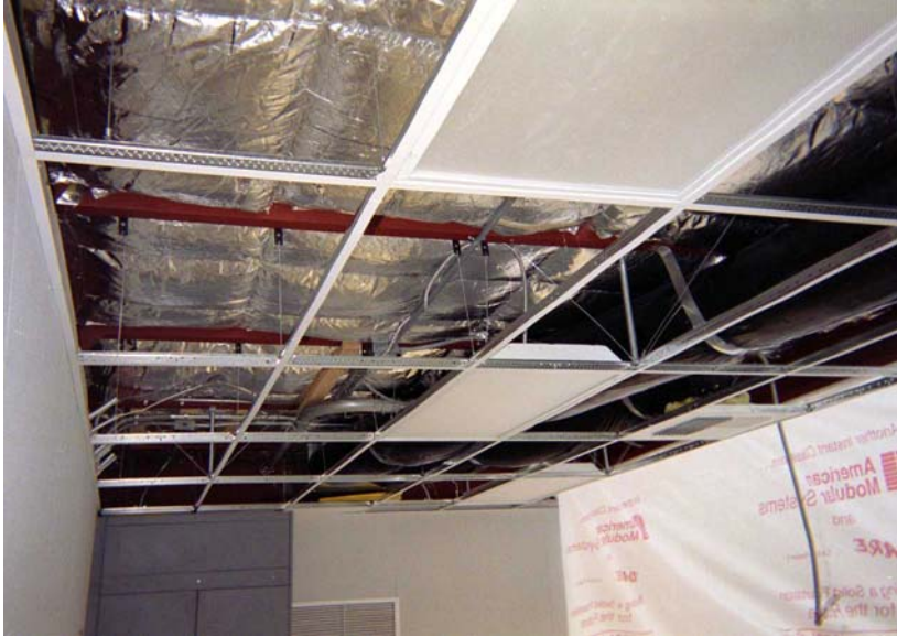
Figure 1: Photograph of the foil vapor barrier provided with roof insulation for the four HPCBS Element 6 RCs.
