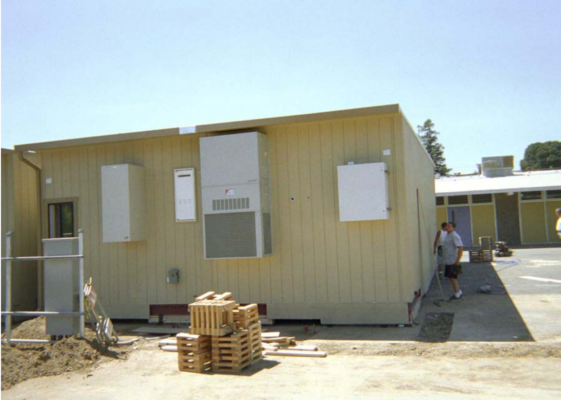
Figure 3: Photograph of the back walls of joining modules for a HPCBS Element 6 RC, each with mounted components of the standard or IDEC HVAC system.
