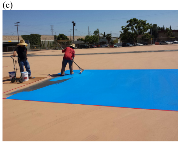
112 Figure 2. Image (a) is the proposed design of the Gardena Elementary School cool schoolyard and image (b) shows 113 the pre-existing blacktop area that was coated in the summer of 2013. Image (c) was taken during the application of 114 the cool coating and image (d) shows the completed project. Sources: Los Angeles Unified School District and 115 Streetbond 2013.
