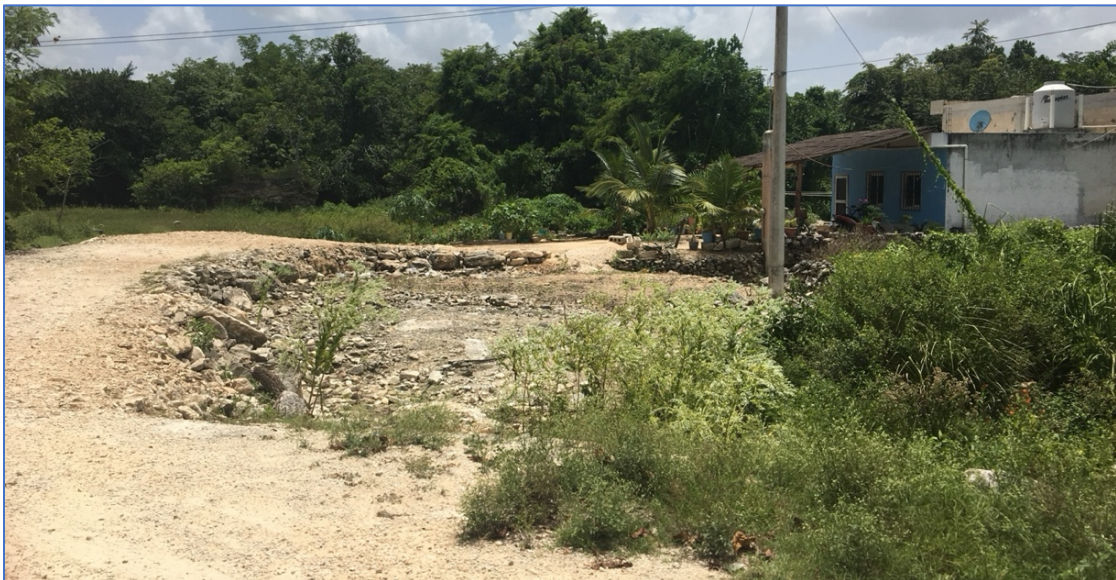
Figure 9.2 Completed road in 2019 Cobá.
