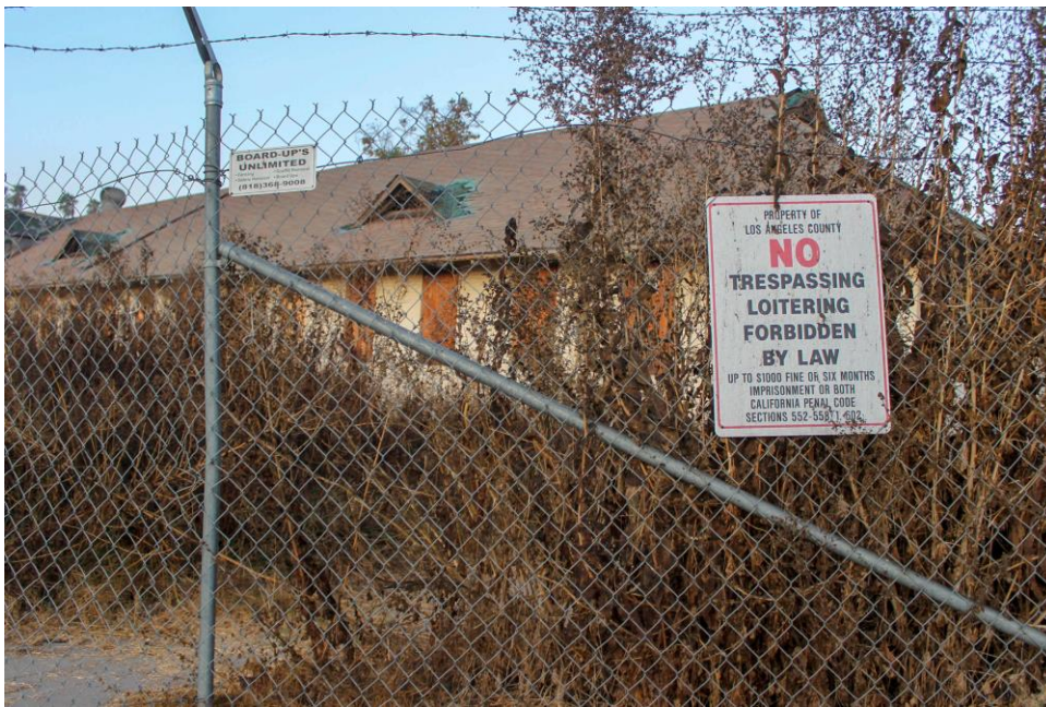
Figure 2.6: Old Rancho boarded-up infirmary. In the foreground, the image shows a “No trespassing sign” hanging on a barbed wire fence. In the background, behind the fence, an old, decaying building with the windows boarded up sits among dead, overgrown weeds. Photo by author.
