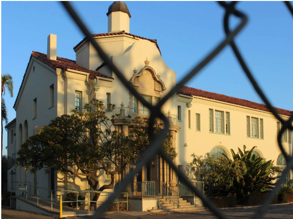
Figure 2.8: Fenced in Old Rancho administration building. In the image, A chain-link fence obscures the view of a building, with the year of its construction, 1926, mounted on a grand entryway. The building is white with deep red roof tiles, built in the Spanish Colonial Revival style. Well-manicured plants adorn the front entrance. Photo by author.
