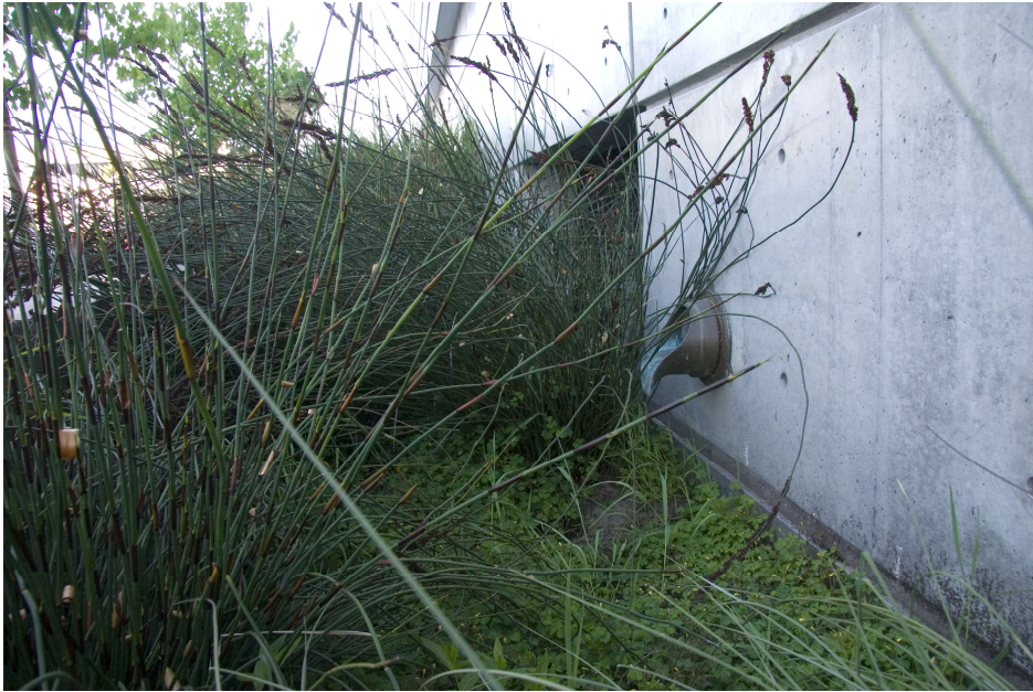
Emeryville Station East, Emeryville
