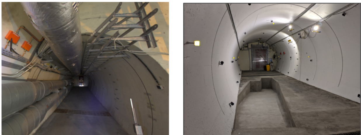
Figure 3.3: TI12, before (left) and after (right) civil engineering intervention [10].
