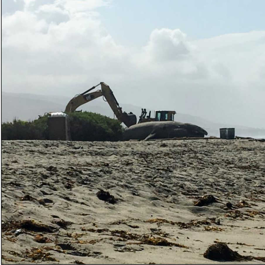
Photograph 3.2: A hydraulic excavator begins dismembering Gray’s tale.
