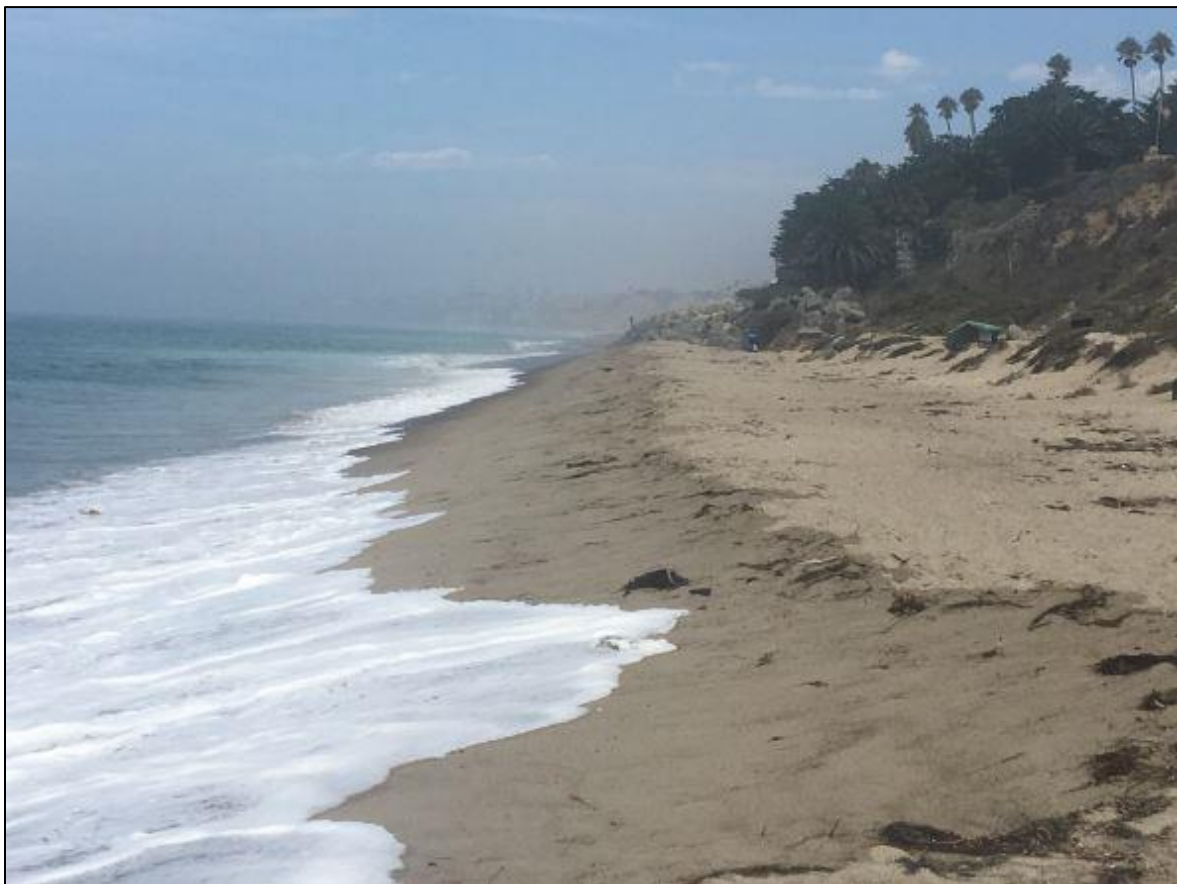
Photograph 1.11: A 5.9-foot high tide on September 19, 2016, inches closer to the banks of the railroad tracks passing through San Onofre State Beach.
