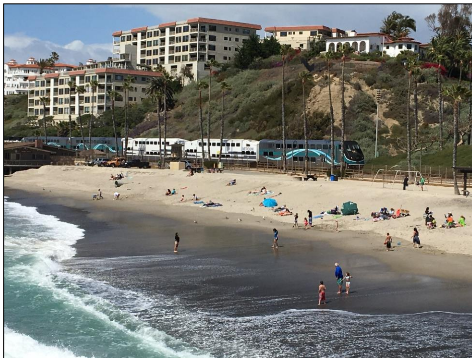
Photograph 4.5: A view of the rising sea level between the Pacific Ocean and Surfliner train tracks in April 2016.
