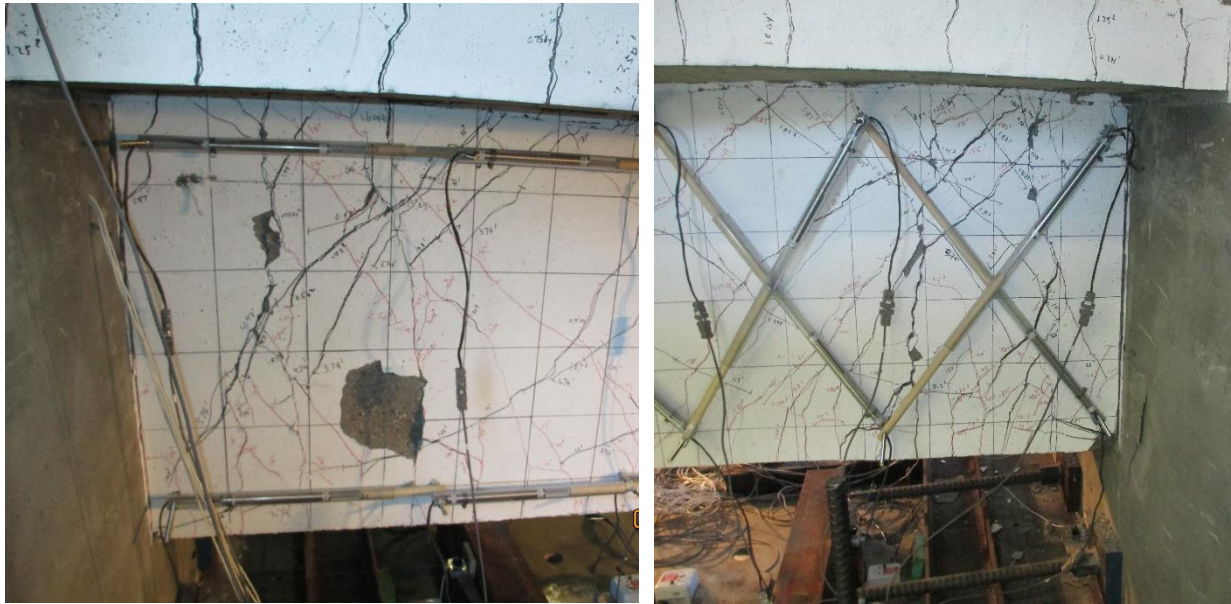
Figure 5.29: Cracking pattern at the fixed end at 3.0% drift on both sides of beam
