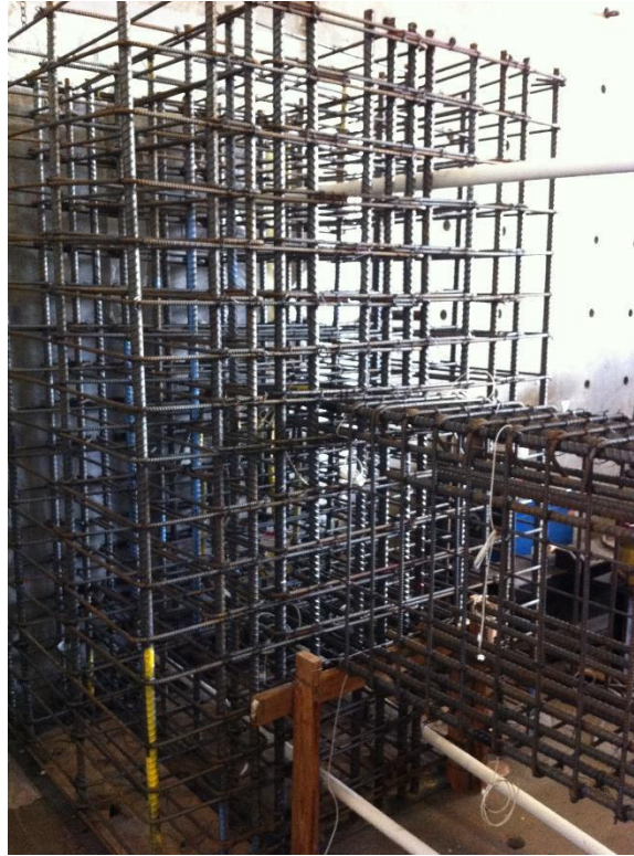
Figure 4.15: Photograph of completed reinforcement for reaction block
