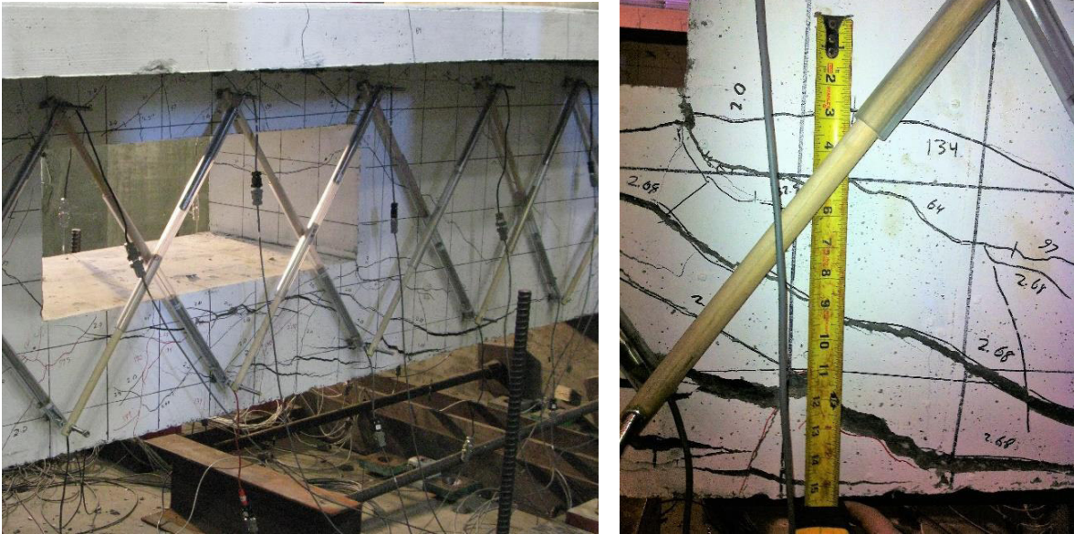
Figure 5.6: Left: Widening of flexural cracks at 3.0% drift; Right: Crack were approximately 5/8-1.0-inch wide
