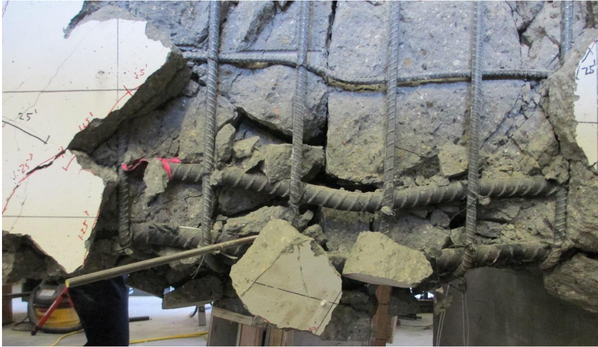
Figure 5.31: Buckling of bottom bars for S4
