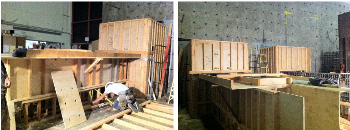
Figure 4.6: Almost completed formwork for S4
