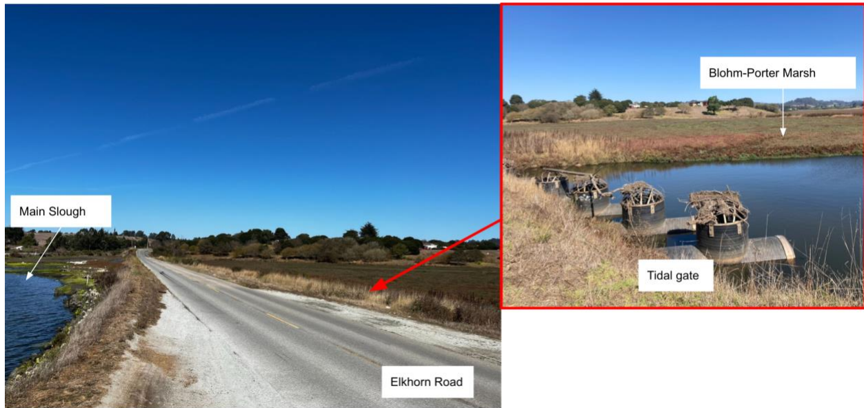
Figure 6. Tidal gate at Elkhorn Road separating the Blohm-Porter Marsh Complex from the main Elkhorn Slough channel. The Blohm-Porter Marsh Complex is at a noticeably lower elevation than the land on the other side of the road by the slough channel.
