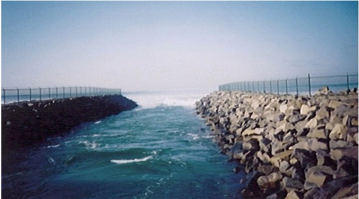
Figure 5-19. Outlet jetties for Agua Hedionda Lagoon that create the surfing break “Warm Water Jetties.”
