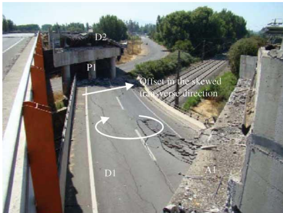
Figure 2.2 One of the many skew bridges that collapsed during the 2010 Maule, Chile, Earthquake seen on the right. The nearby bridge (partially seen on the left) that had straight abutments survived (Kawashima et al. , 2011).
