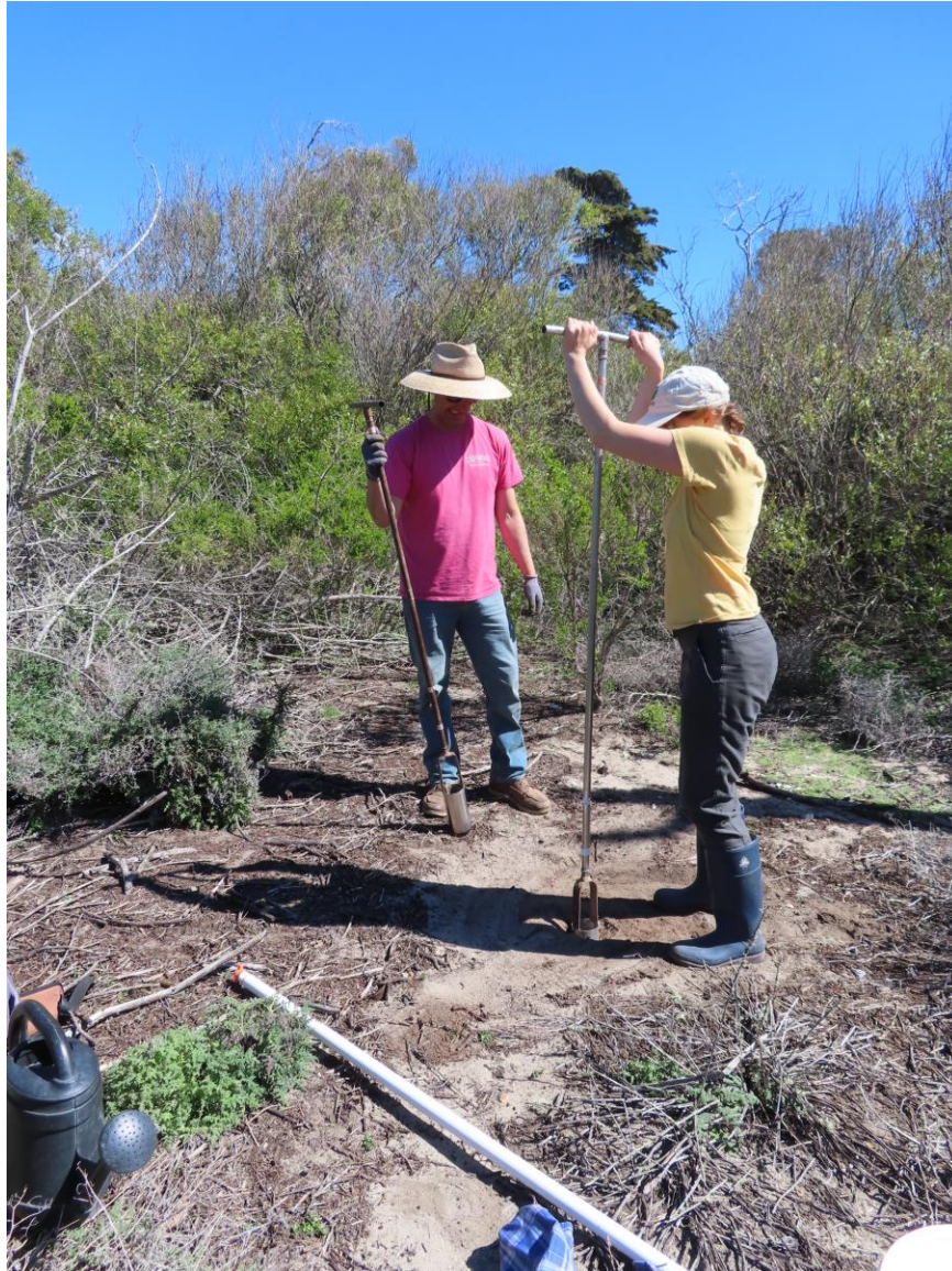
A photo showing installation of the West Main Channel index well at plot 5.
