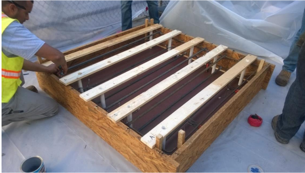
Figure 2-12: Reinforcing Steel Layout for Slab Prior to Pour
