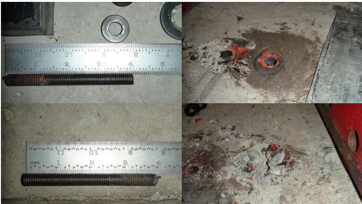
Figure 4-10: N2 Failure Photographs for A3 Anchor (top left) and Concrete Surface (top right) and A4 Anchor (bottom left) and Concrete Surface (bottom right) for BBM Test Sequence
