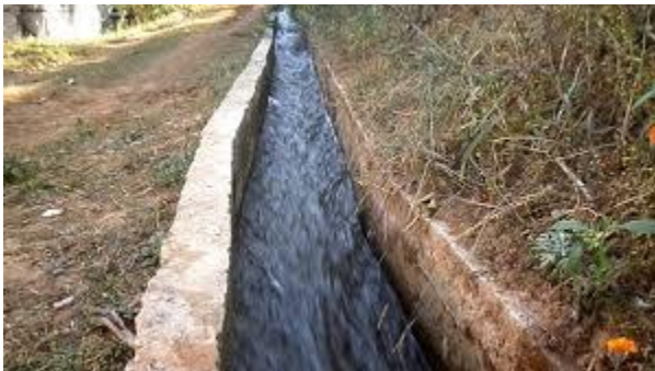
(Figure 1.7 depicts a surviving canal that channels spring water into reservoir ponds, pits and hiti )
