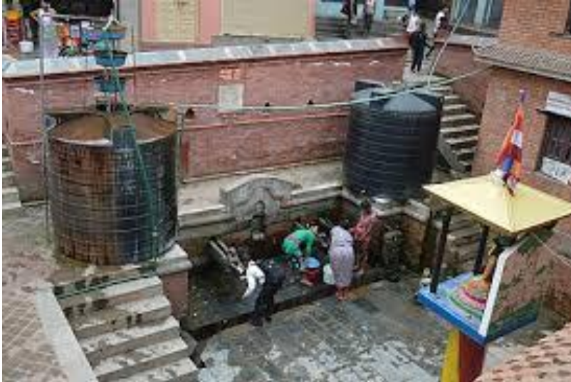
(Figure 2.5: Residents of the historic Newari city of Bhaktapur collect water from an ancient hiti. Plastic tanks and PVC pipes have replaced the historic canal system here, due to damage during road construction)
