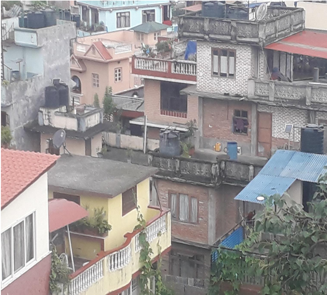
(Figure 2.4: Black 1000-liter water storage tanks are seen on rooftops of houses in a dense urban neighborhood)
