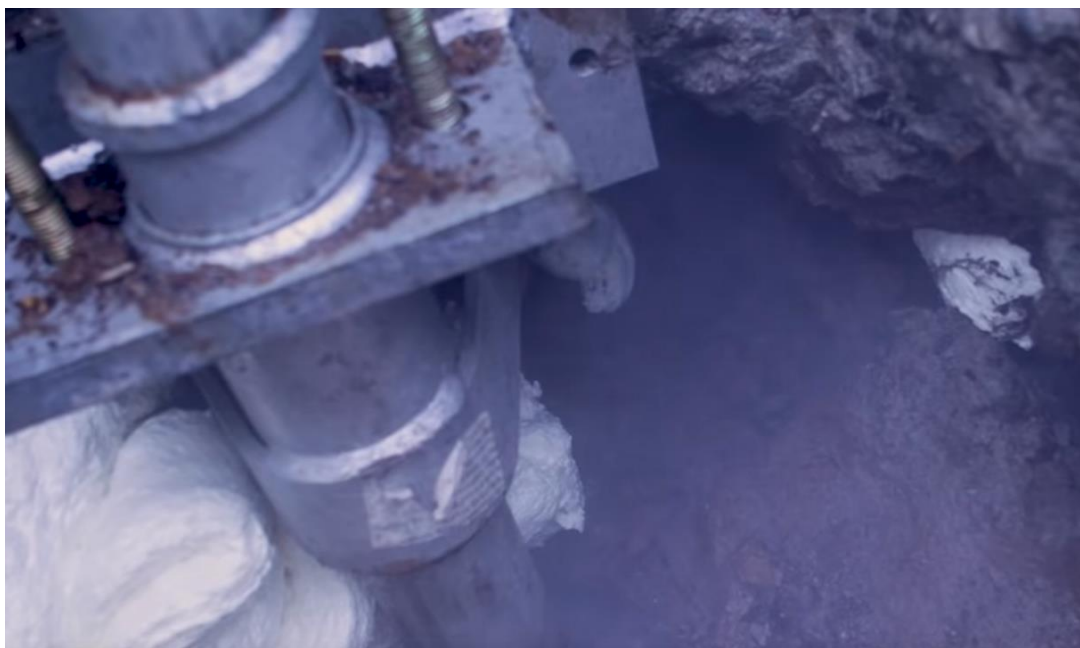
(b) Injection of the expansive polymer under the structure.
