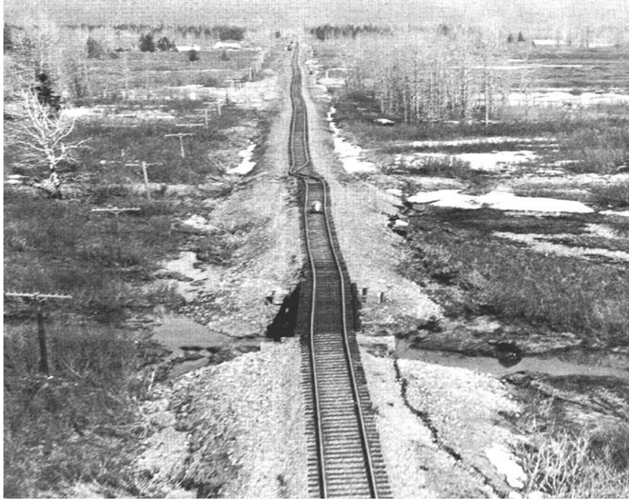
(a) Railroad embankment during the 1964 Alaska earthquake
