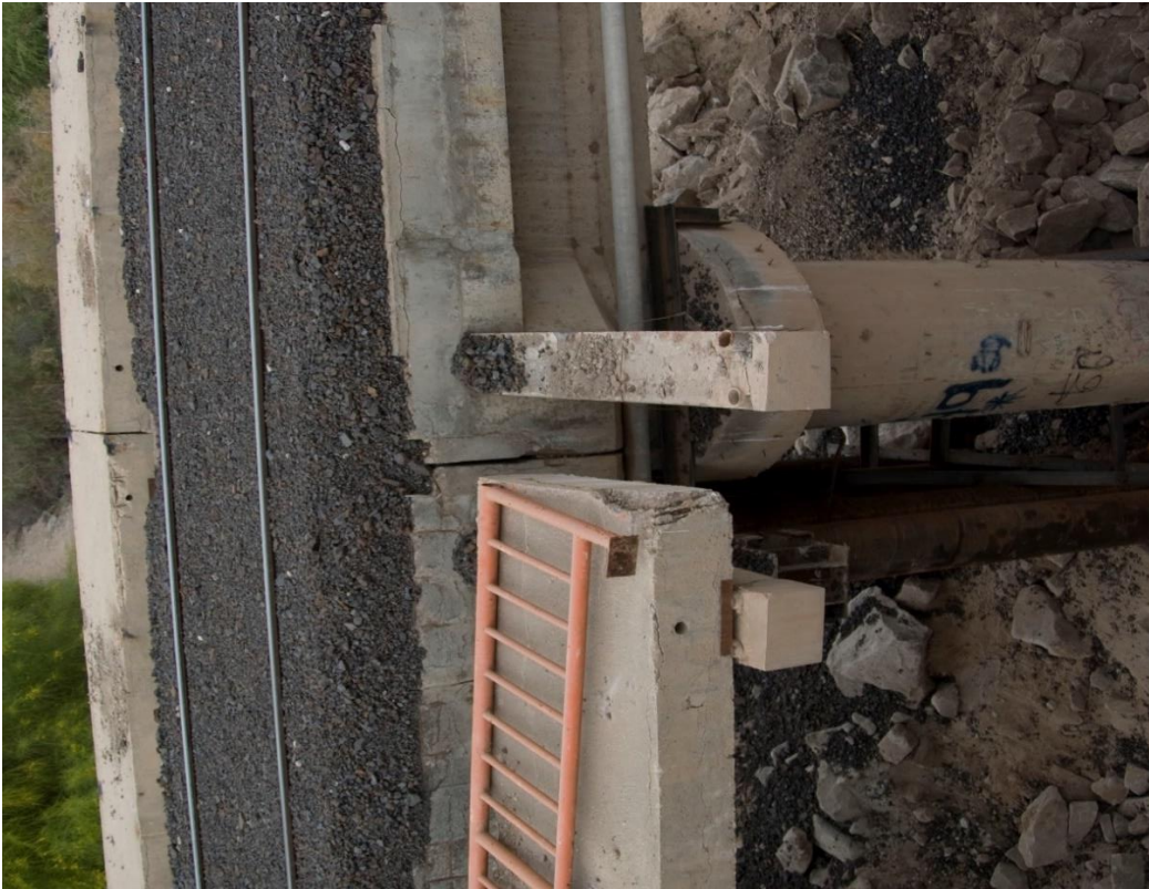
(a) Nearly unseated Span at Bent B2 of Railroad bridge (b) Unseated Span at Bent B5 of Railroad bridge
