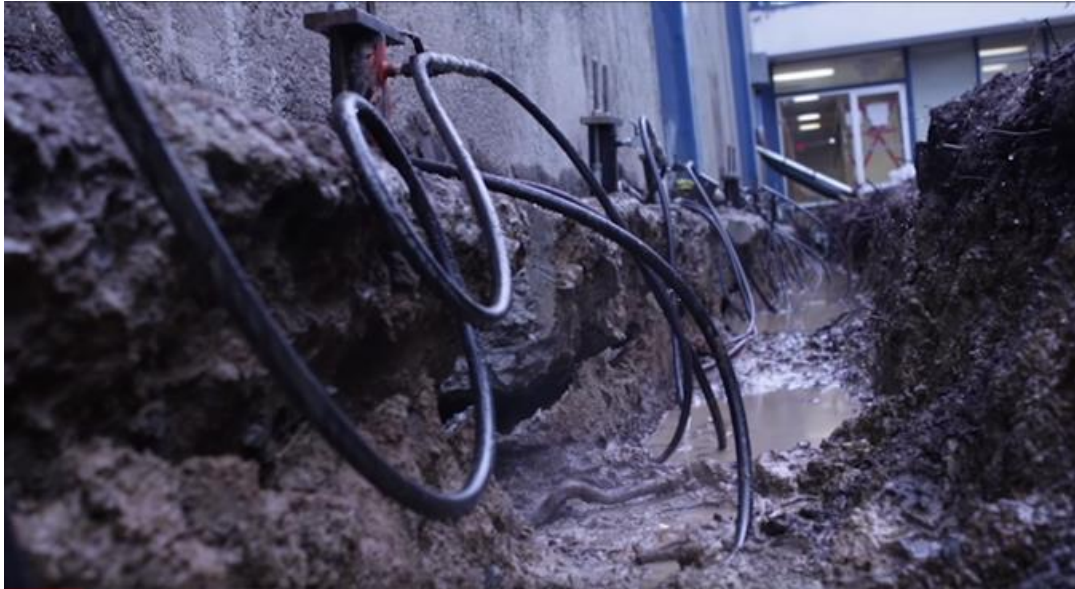
(a) Shoring the perimeter of the structure prior to polymer injection
