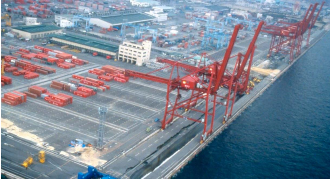
(a) Lateral spreading induced damage to a pier and cranes during the 1955 Kobe earthquake
