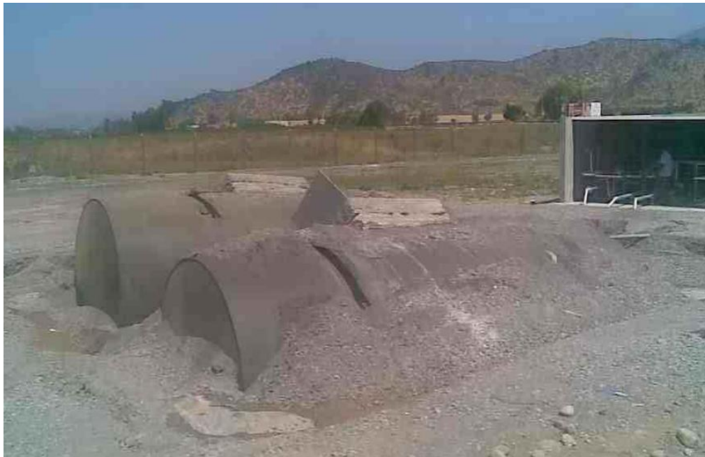
(b) Buoyant rise of an underground tanks from the 2010 Maule earthquake, Chile
