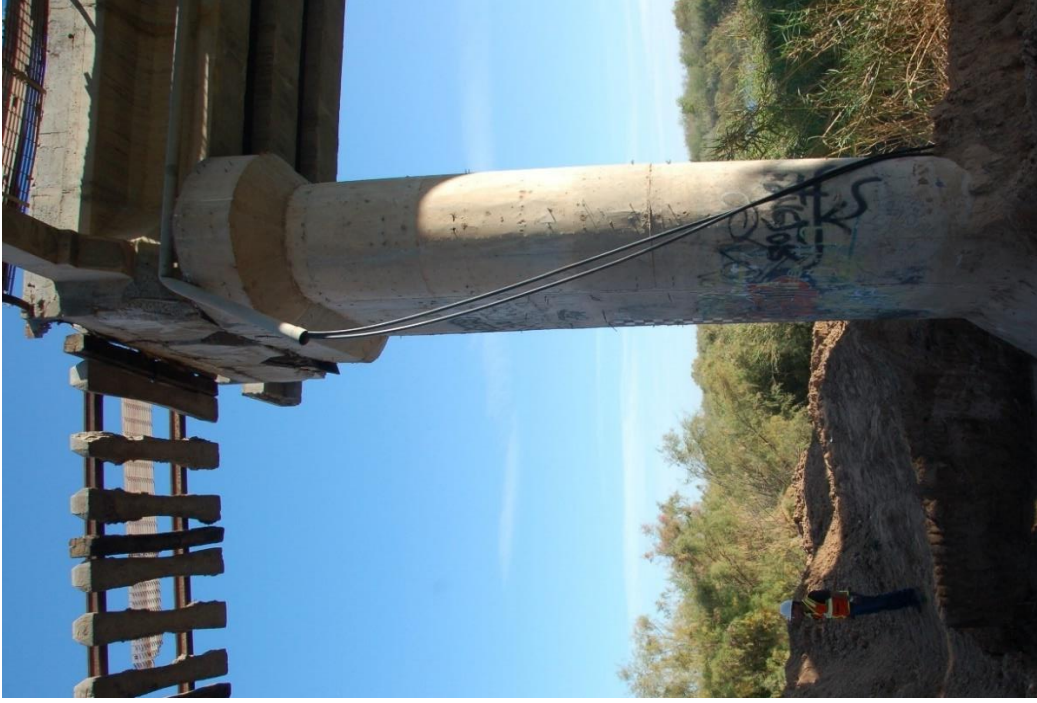
(a) Nearly unseated Span at Bent B2 of Railroad bridge (b) Unseated Span at Bent B5 of Railroad bridge
