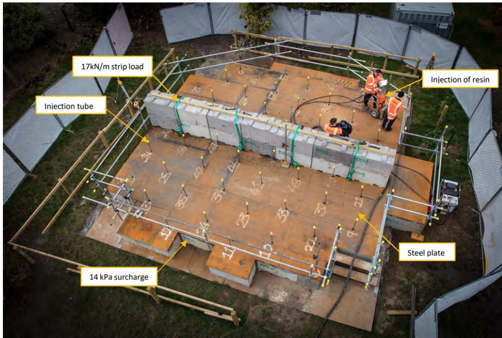
(a) Polymer injection test panels at the red zone site (site 3)
