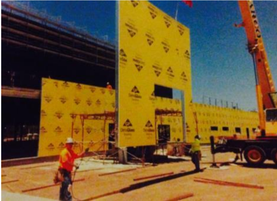
Figure 9: Prefabricated Exterior Wall Panels 18
