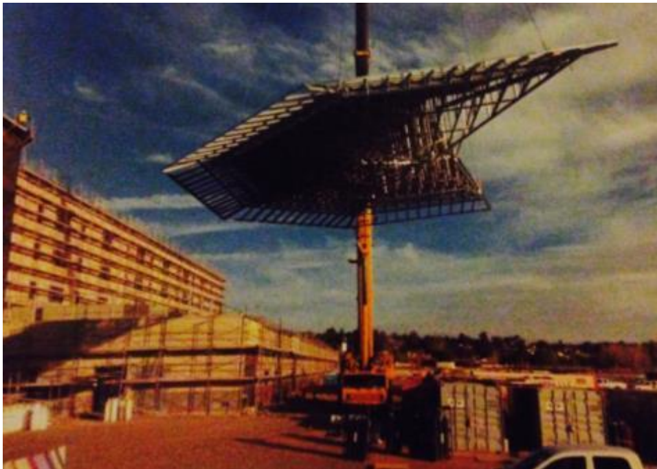
Figure 10: Prefabricated roof truss
