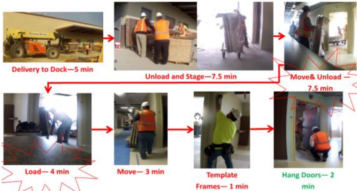
Figure 11: Design of door installations
