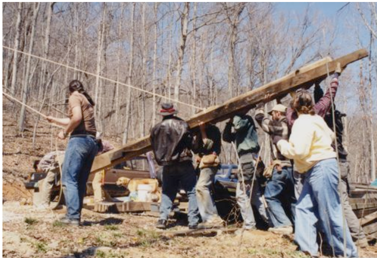
Figure 3.9. Raising a timber-frame house at a work party.
