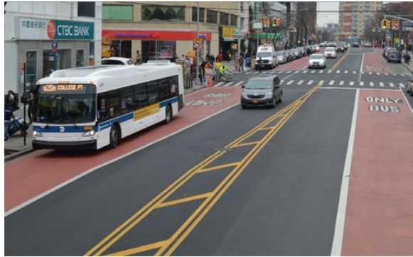
New York City - Queens Two-Way Bus Lanes speed up transit service in congested roads Source: StreetblogNYC
