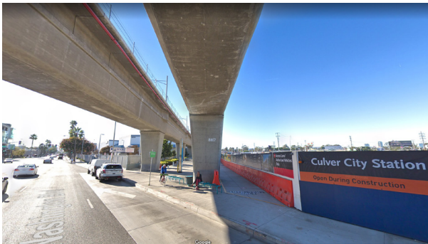
Figure 25. Expo Station - Washington Blvd Entrance
