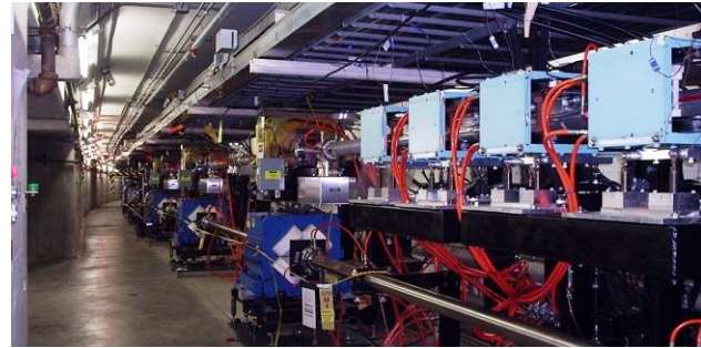
Figure 4. Chicane dipole magnets (Right) installed in the LER (upper beam pipe) for electron cloud tests.
