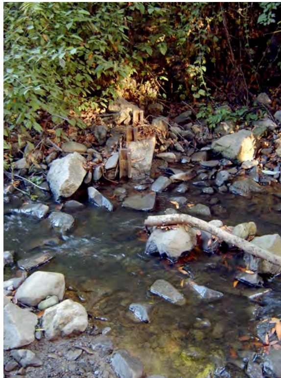
Remnants of removed debris rack
