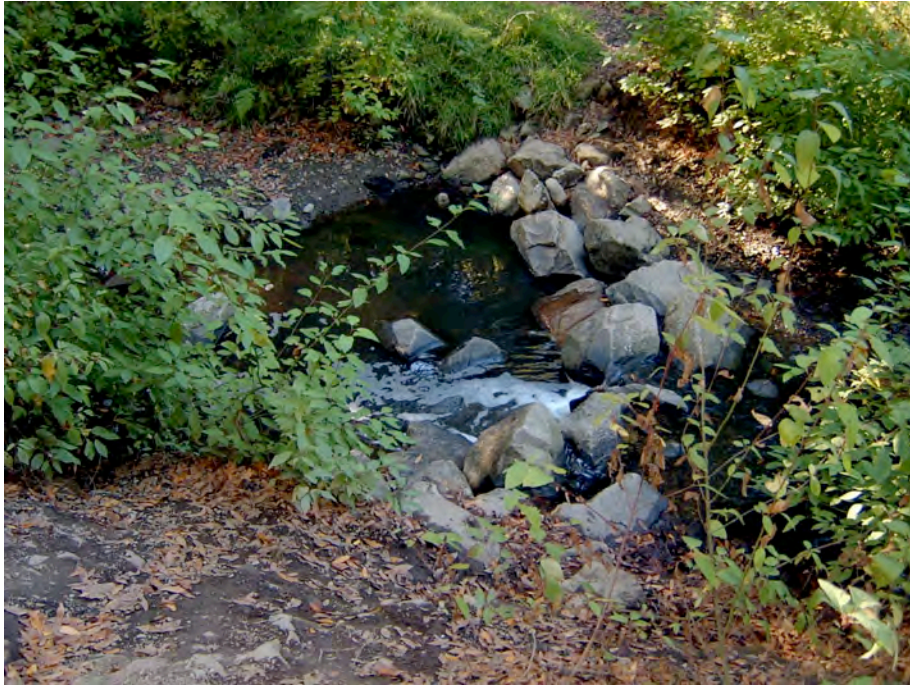
Constructed Rock Weir
