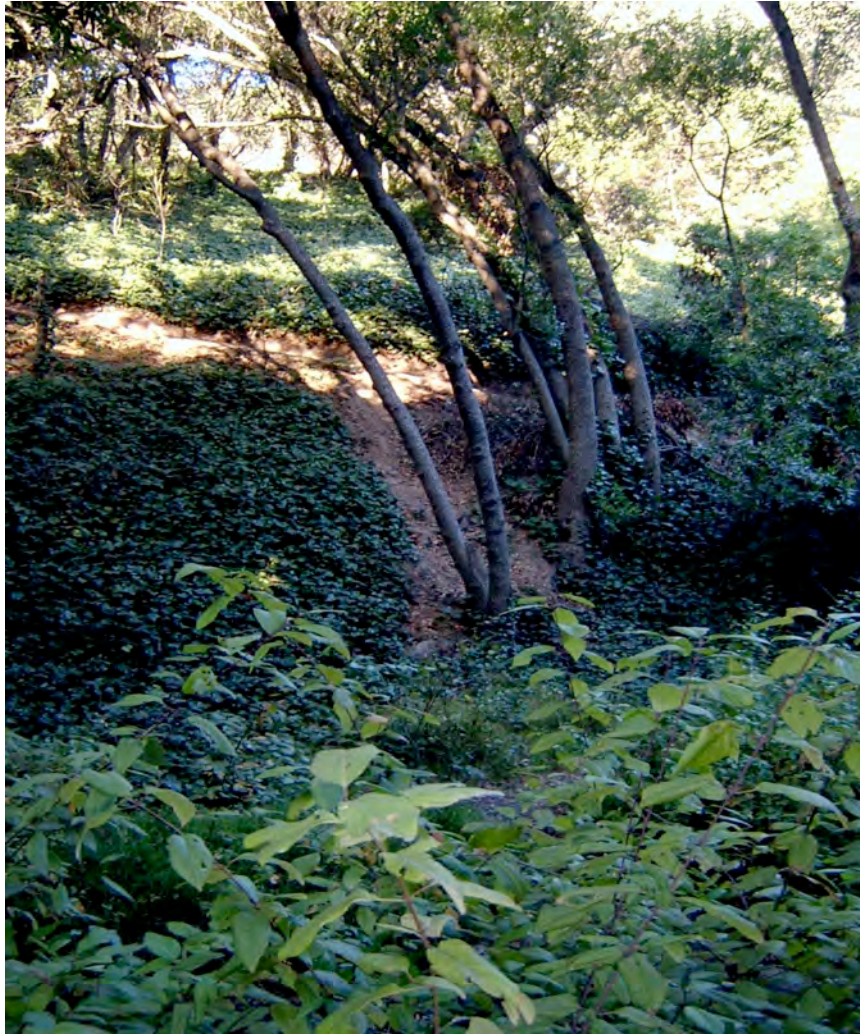
Figure 28: Erosion due to informal creek crossing at rock weir
