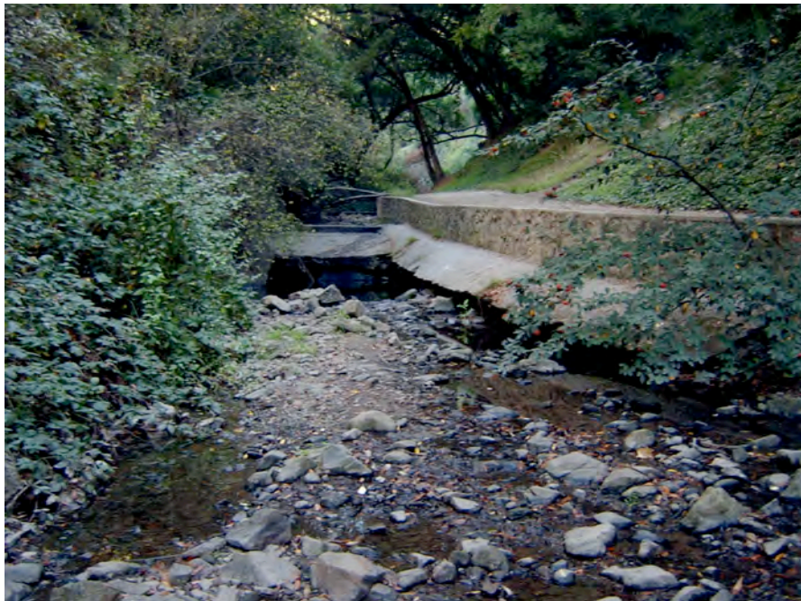
Channel Incision and Upstream Check Dam
