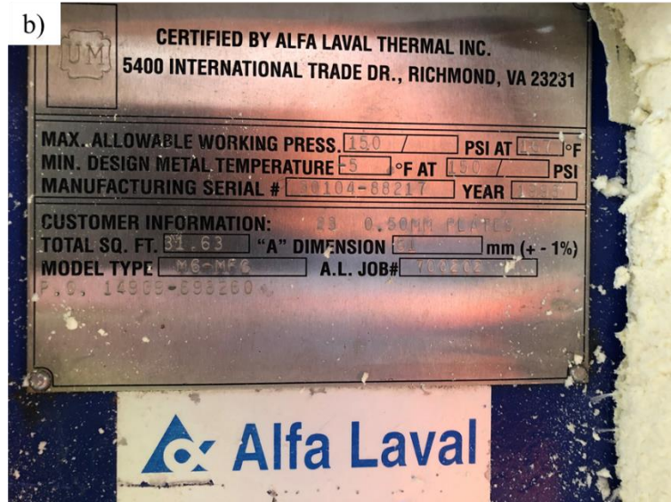
Figure S7. Photo of the plate heat exchanger for energy recovery. a) Heat exchanger on the unit before insulation was added. b) manufacture's information plate.
