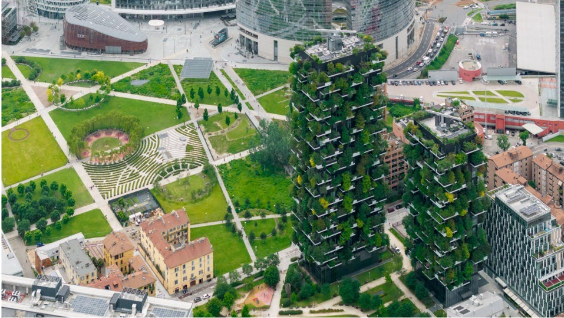
Figure 4. The Bosco Verticale towers with the adjacent Biblioteca degli Alberi Milano park. The image illustrates the lush greenery enveloping the towers and the integration of the adjacent public green open space in the Porta Nuova district of Milan. Photo by Iwan Baan. Featured in Tom Ravenscroft, “Bosco Verticale,” Dezeen, January 20, 2025, https://www.dezeen.com/2025/01/20/bosco-verticale-stefano-boeri-21st-century-architecture/ .
