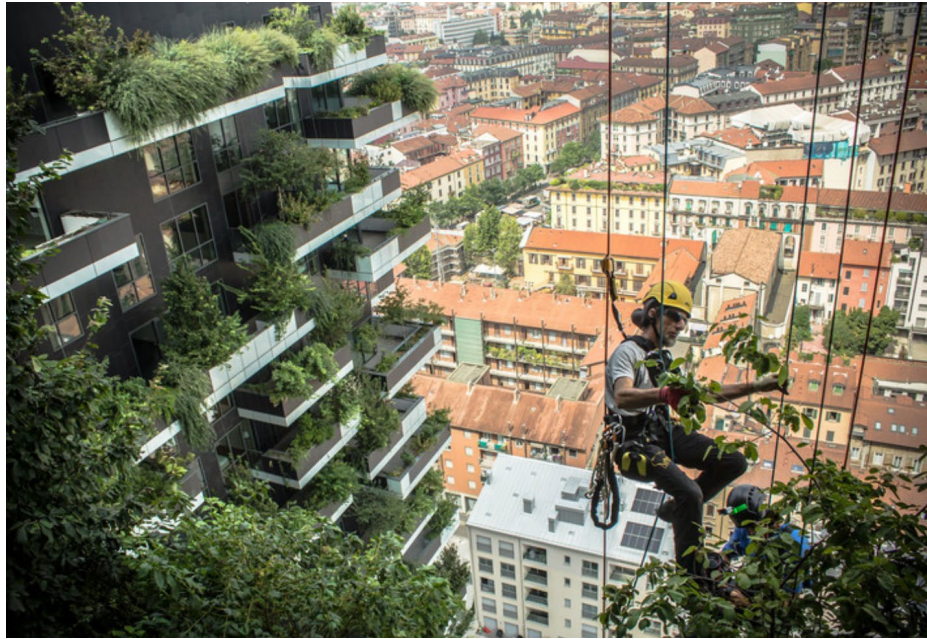
Figure 7. Sky gardener performing routine maintenance on the vertical garden system at Bosco Verticale, Milan. Photograph by Laura Cionci, published October 9, 2015, Milan. From Domus, https://www.domusweb.it/en/video/2015/10/09/the_flying_gardeners.html .
