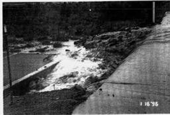
Storm water flowing into inlet structure
