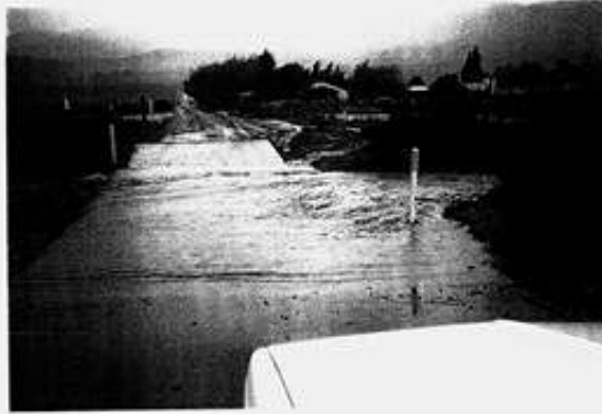
1-16-93 Hennessey Creek storm water flowing south over Reservoir Lane
