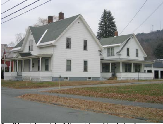
Small lot eight-unit building with parking behind (#7918)
