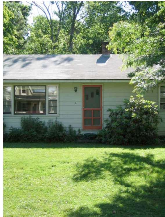
A neighboring house feels closed off from the street
