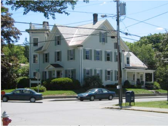
Building & site orient to both sides of street corner (#3748)
