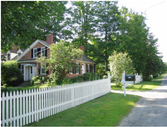
Verge/ROW line marked by picket fence on Main N1 (#4493)
