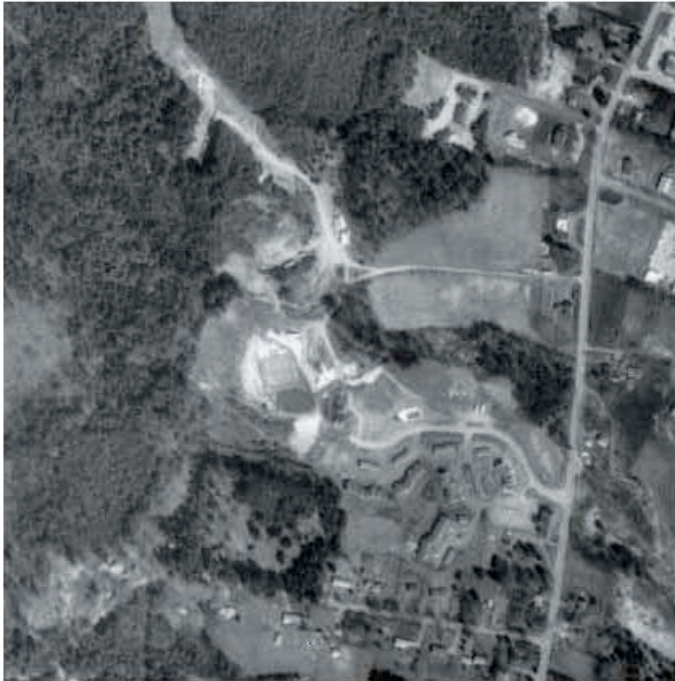
Figure 6-4 Ortho-photograph (1996) with Iris Way in N7 Under Construction
