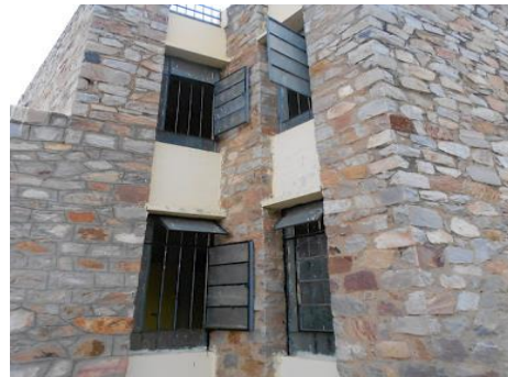
Figure 16. Brick wall coated with stone.
