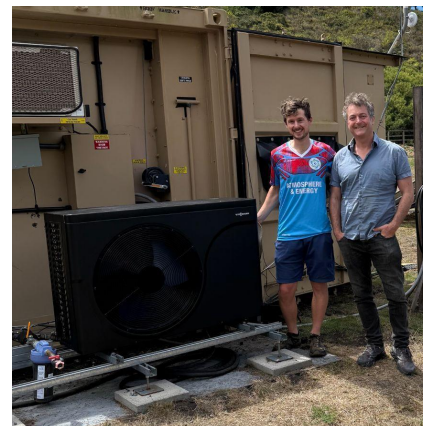
Figure 1: Indoor view of the structure (left) with thermal energy storage and controls systems and fan coil unit; and outdoor view (right) with HP unit. Note the default PTAC unit (through wall) that the experimental HP TES replaces.
