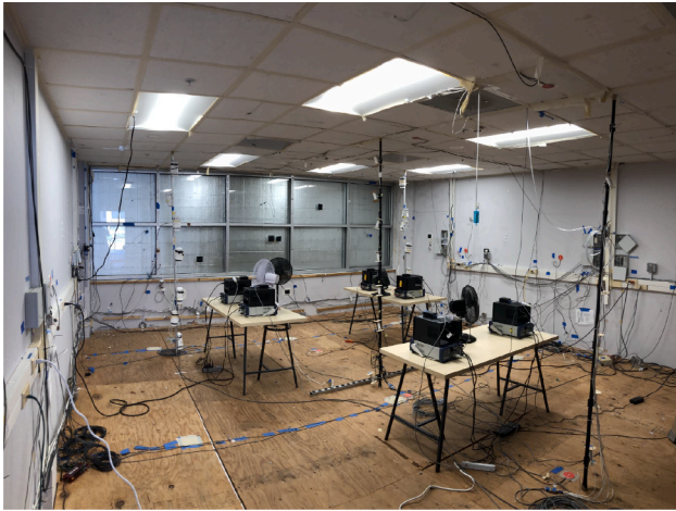
Fig. 6. Test cell experimental setup for AC and DC experiments. Photograph by Jordan Shackelford, LBNL; used with permission.
