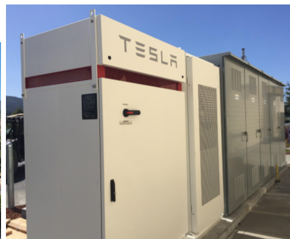
(b) 174 kWh local energy storage capacity with a peak output of 109 kW
