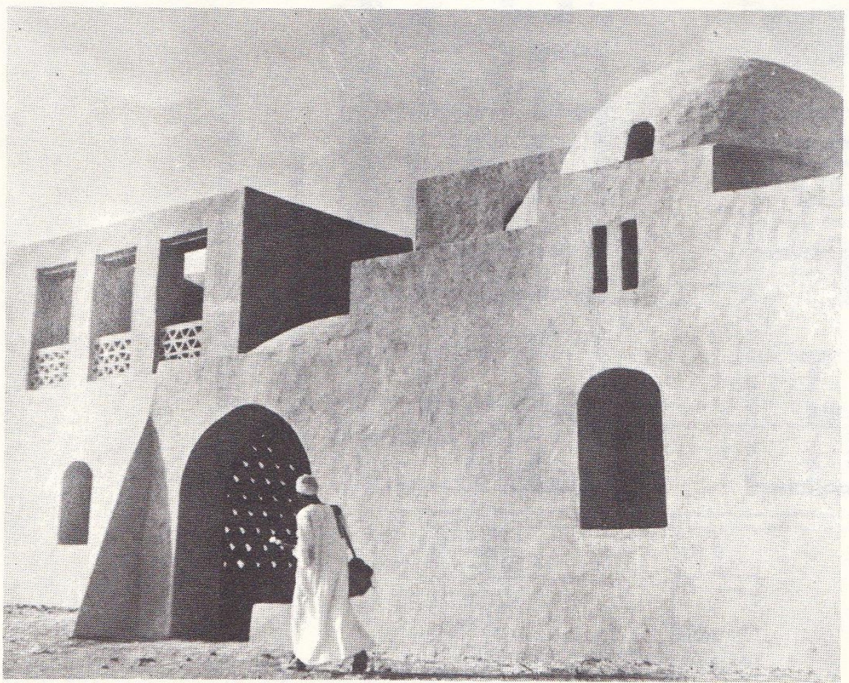
Figure 3.9 Mudbrick houses in new Gournah, 1948. From: Hassan Fathy, Architecture for the Poor (Chicago and London: The University of Chicago Press, 1973)
