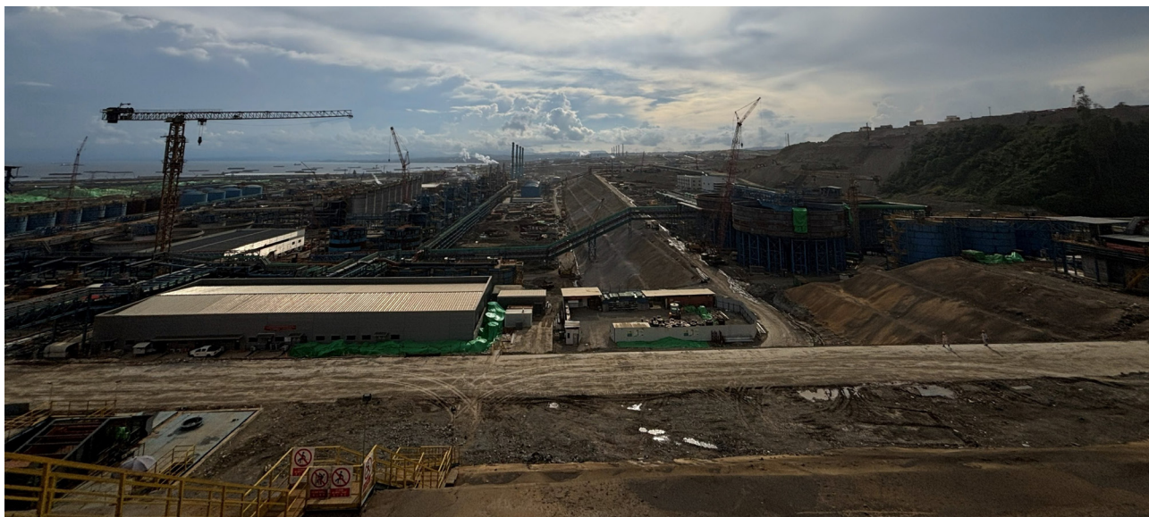
Figure 1: PT Indonesia Weda Bay Industrial Park, one of the largest battery-precursor processing facilities. Source: Author
