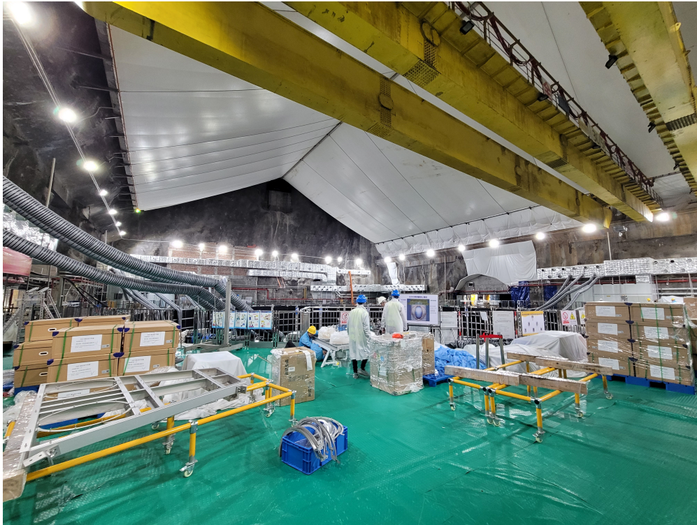
Figure 5.11: Top of JUNO experimental hall with yellow crane rails pictured along the ceiling.
