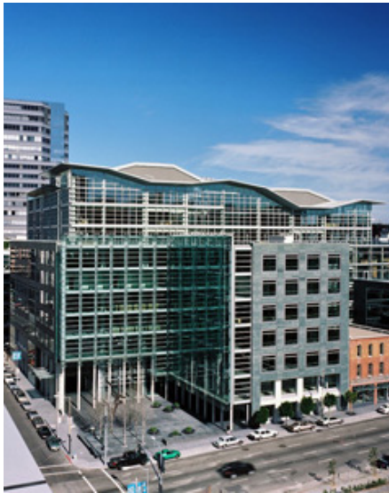
Figure 43: 405 Howard St. building
