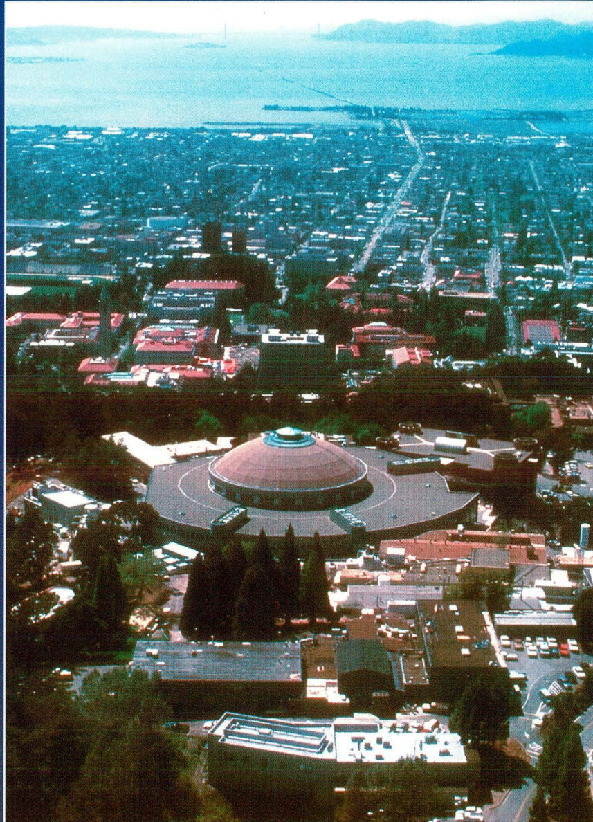
The Advanced Light Source is situated in the hills of Berkeley, California, overlooking the San Francisco Bay. Its building incorporates the dome that once housed the 184-Inch Cyclotron built by Lawrence Berkeley Laboratory's founder E.O. Lawrence.
