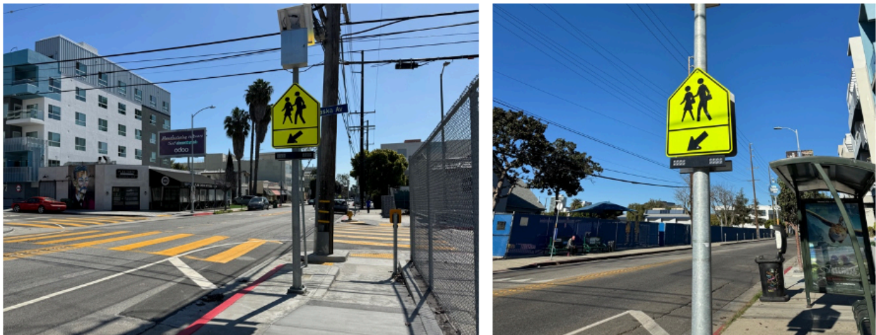
Figures 14 - 15. Crosswalk Conditions
