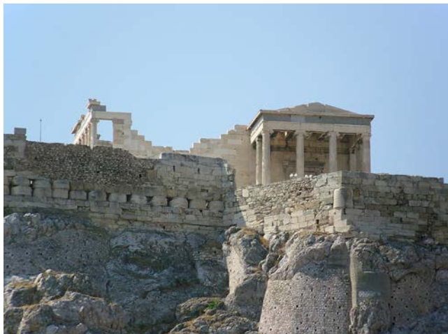
Figure 3.2. Visible on the north slope of the Athenian acropolis, just below the Erechtheion, is a row of column drums. These were originally intended for use in the "older Parthenon," which was not yet finished at the time of the Persian sack in 480 B.C. Only later were its remains built into the defensive curtain wall of the acropolis (Courtesy Eusebius [GuillaumePiolle]).
