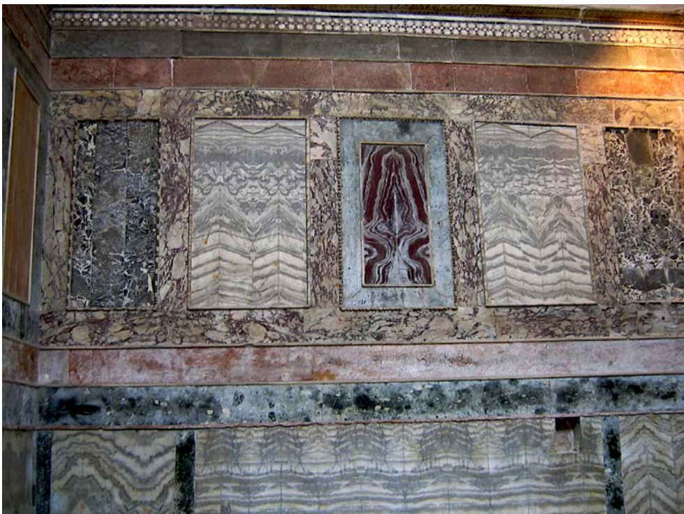
Figure 17.4. Book-matched pattern on a revetment in the naos of the church of the Chora, Constantinople, 12 th /14 th century.
