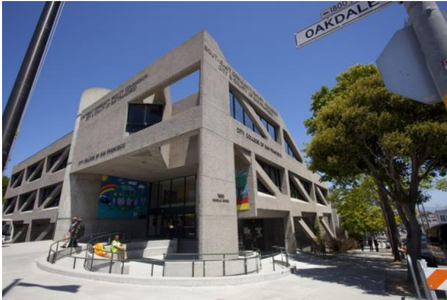
Figure 12. The Southeast Community Facility built under the 1986 Mitigation Agreement.
