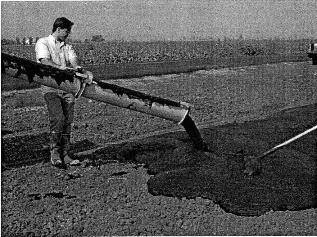
Figure C.8: Application of SLD sediments to FP-1 using cement-truck chute (10/21/99).
