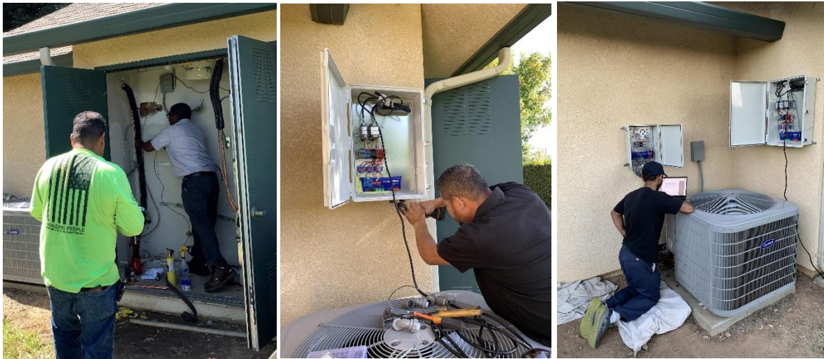
Figure 4. Instrumentation installation and wiring
