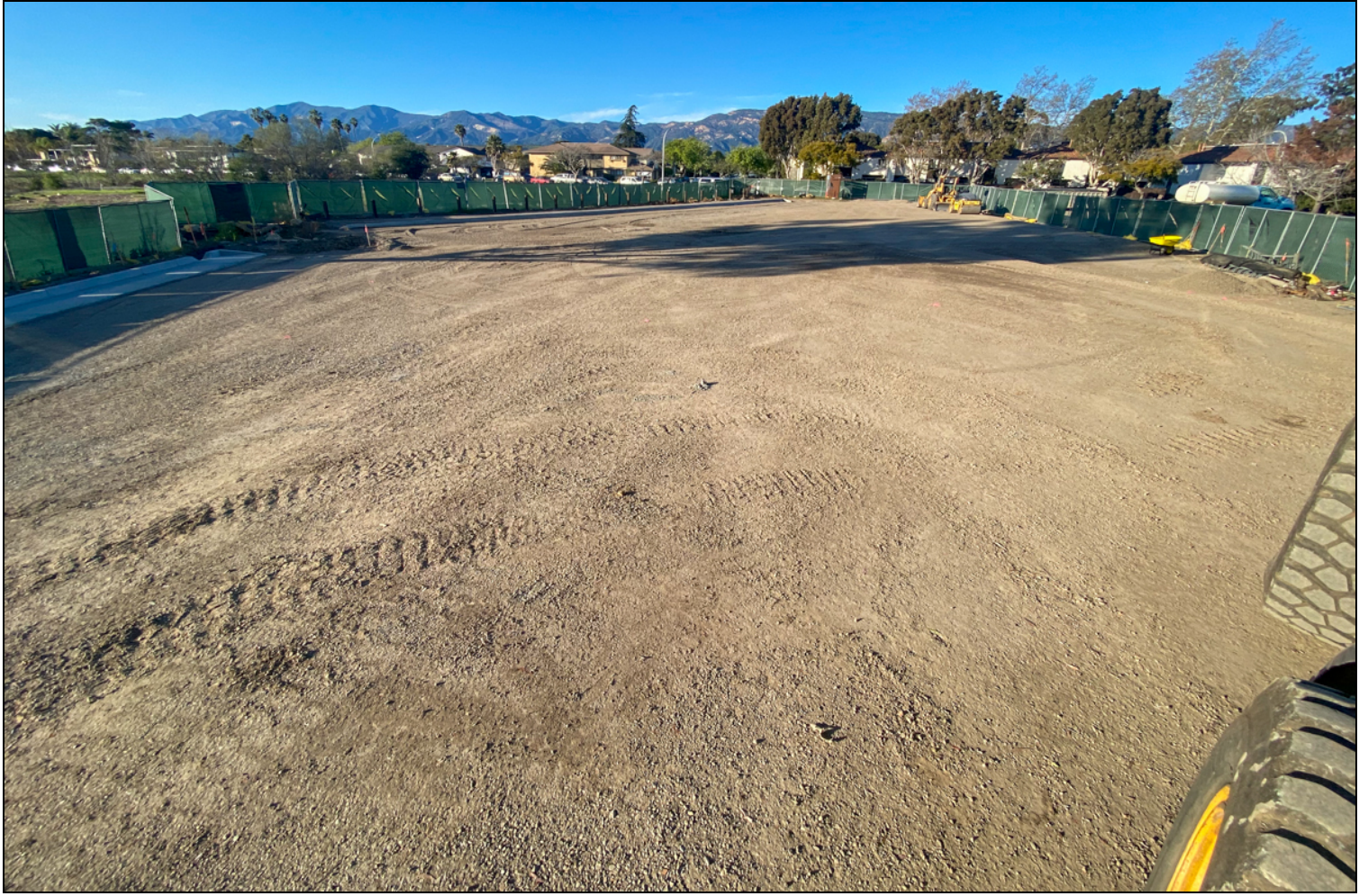
Newly graded parking lot.
