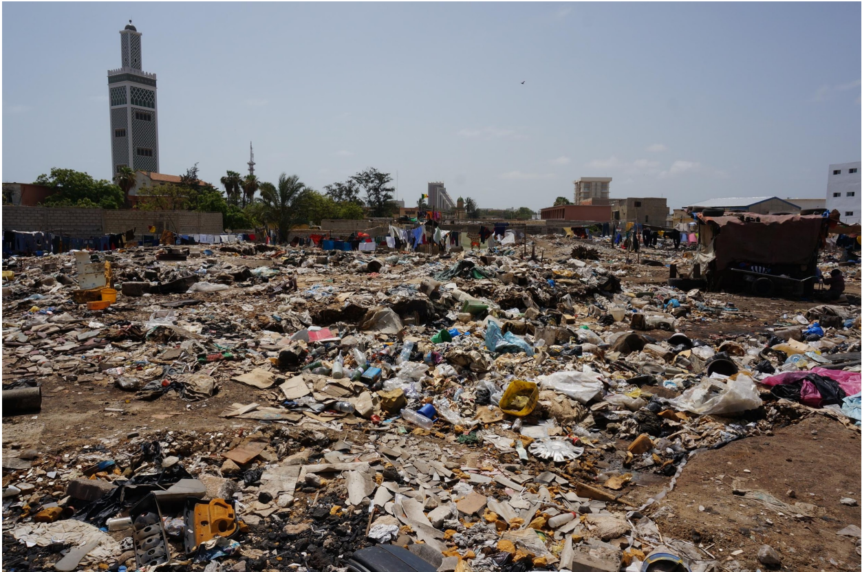
Figure 4.7 Settlement Demolition in Preparation for New Market Building Photo by Author
