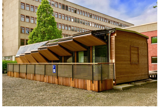
Figure 4. Rooftop building with roof and facade mounted photovoltaic system in Berlin (Germany).
