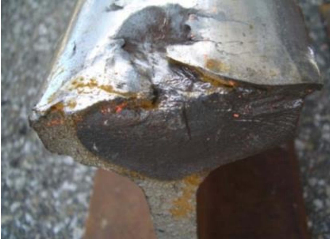
Figure 4-7: Engine burn fracture defect in the rail head (Federal Railroad Administration, 2015).
