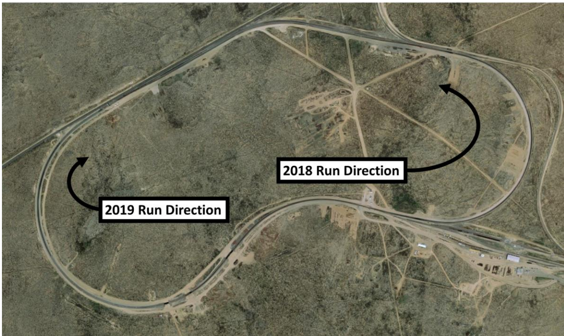
Figure 5-16: Satellite view of the HTL loop used in the 2018 and 2019 field test.
