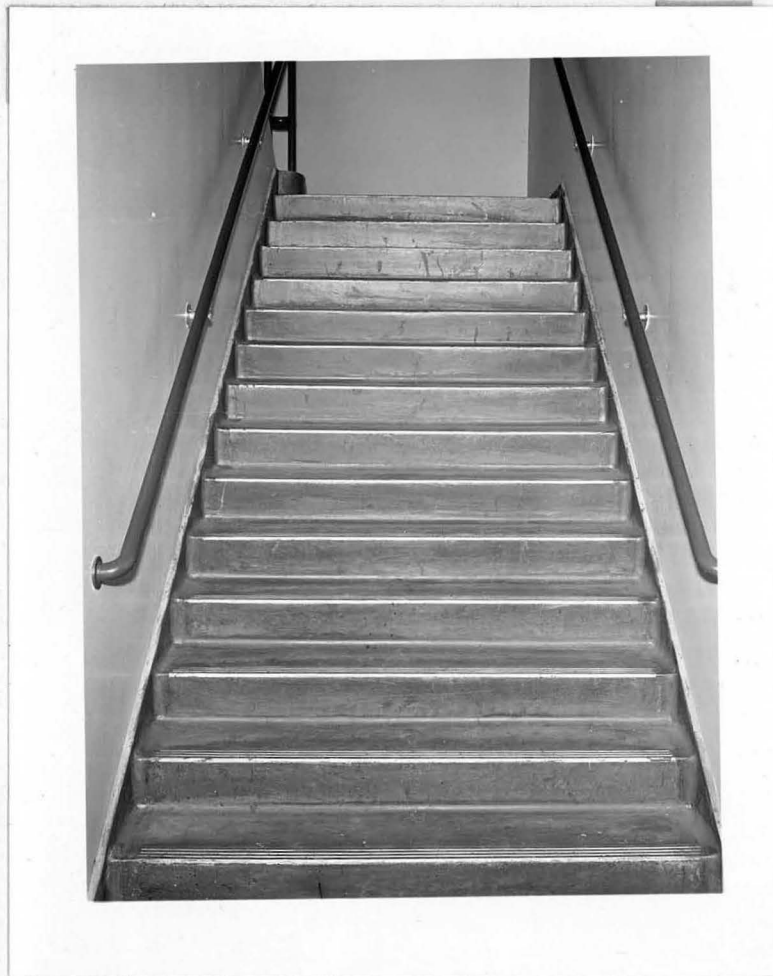
Fig. 2. Treating concrete with paraffin.
